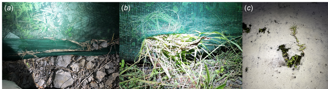
Fig. 4. Issues with design and maintenance of polyethylene amphibian exclusion fence constructed on Kooragang Island, Australia in 2020, to keep Litoria aurea out of a construction zone. (a) Section of fence not buried underground. (b) Horizontal cut in fence material caused by mower blades during vegetation maintenance. (c) Degradation of geofabric material used to line the outside of the fenceline.
