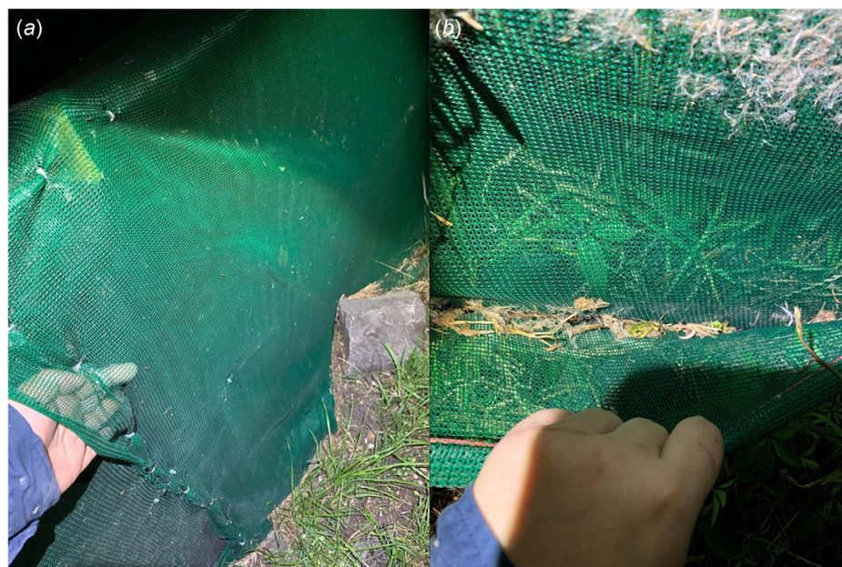
Fig. 1. Design and maintenance issues for polyethylene amphibian exclusion fence on Kooragang Island, Australia installed in 2019 to keep Litoria aurea out of a construction zone. Images show gaps caused by (a) spaces between metal pins used to connect fence sections together, and (b) a tree frog stuck between folds of fence material near the ground.
