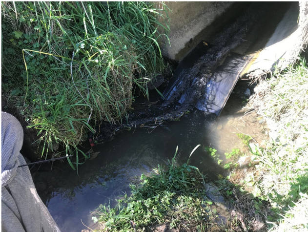
Fig. 1. Rubber ramp and spat rope installed at the outlet of the perched culvert in an unnamed tributary of Oldham Creek, Nelson, New Zealand. Barrier net retaining fish within the test arena is visible to the left of the picture.
