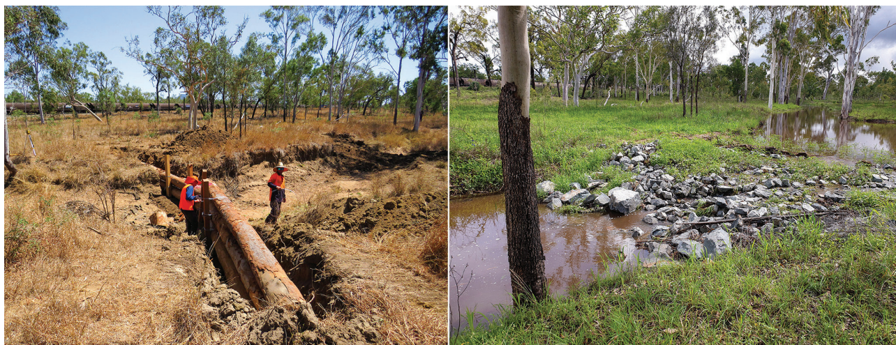
Figure 3: Log weir on the NQ Dry Tropics' demonstration hub in North Queensland.
